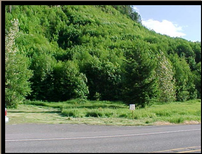
Shared paved access apron
